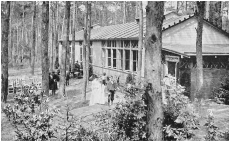
1/ Main building with classrooms Waldschule Charlottenburg 1904
