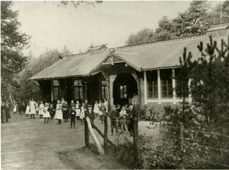
7/ School building Waldschule Mönchengladbach 1906
